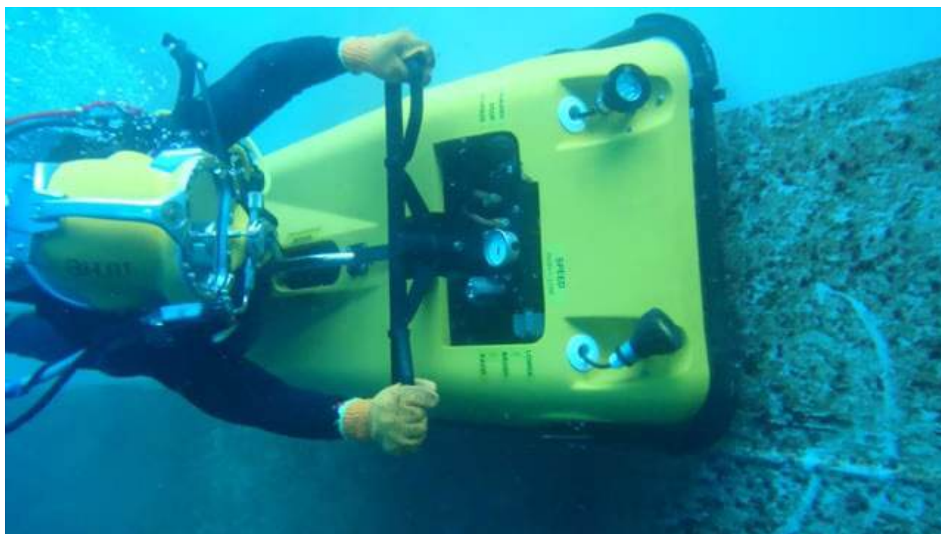
Photo 4: Diver-operated cleaning cart.
